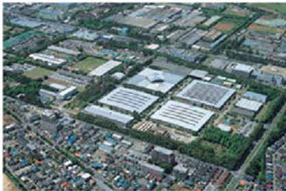
Hitachi Narashino Plant in Japan
